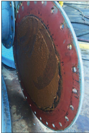
Figure 5: Inside of tank access cover.
