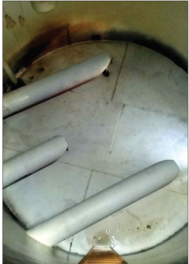
Figure 8: CCW tank floor after water blasting.
