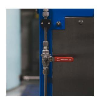
All fittings, valves, and tubing on an Anodamine dosing system are premium grade 316L stainless steel. All piping is standard 1/2" AISI-316L stainless steel with terminations in compression piping fittings.
