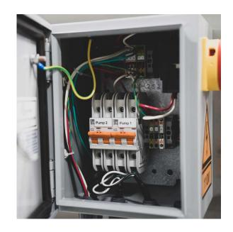
Located on the rear of the dosing system pump frame, this electrical connection box is where main power to the system is wired, featuring a circuit breaker for each pump and controller, along with an electrical disconnect switch that has LOTO-capabilities.
