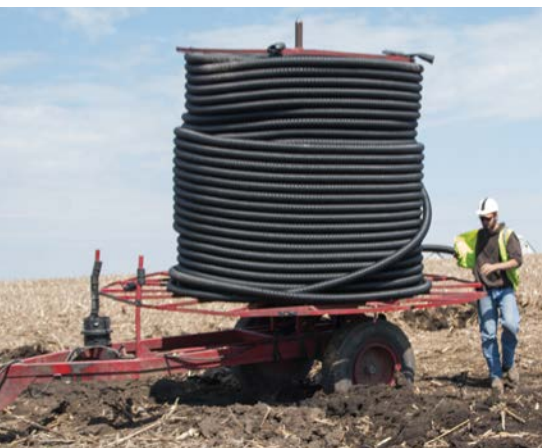
Drain tile is placed in trenches to improve drainage for higher crop yields.
