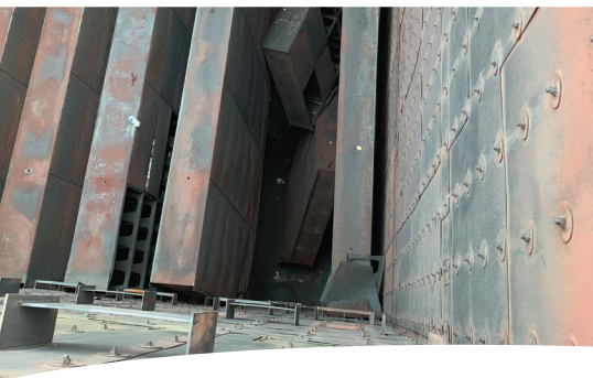
Before photo: failed vertical silencer panels for 501F.
