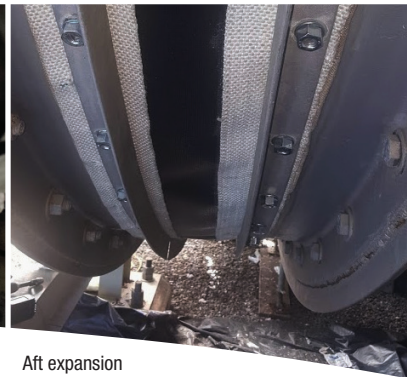
Aft expansion belt upgrade.
