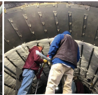
Insulating & installing liner.
