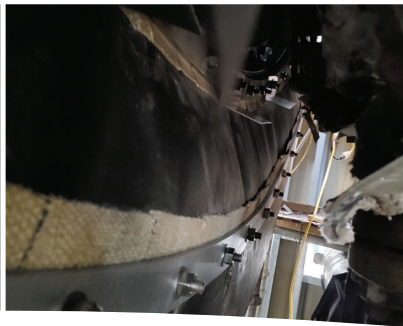
Forward trough expansion joint seal.
