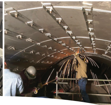
Torquing & tack welding nuts.
