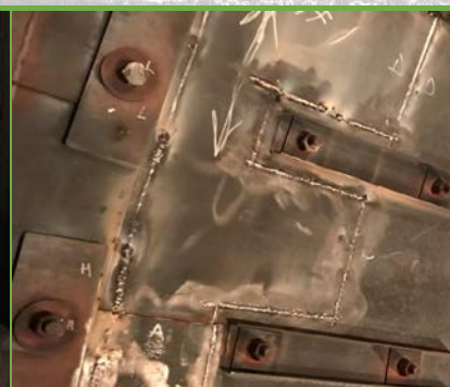
Local "hot spot" repair
