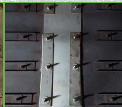
Replace field joints
