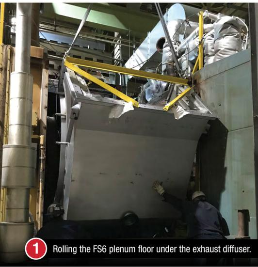
1 Rolling the FS6 plenum floor under the exhaust diffuser.
