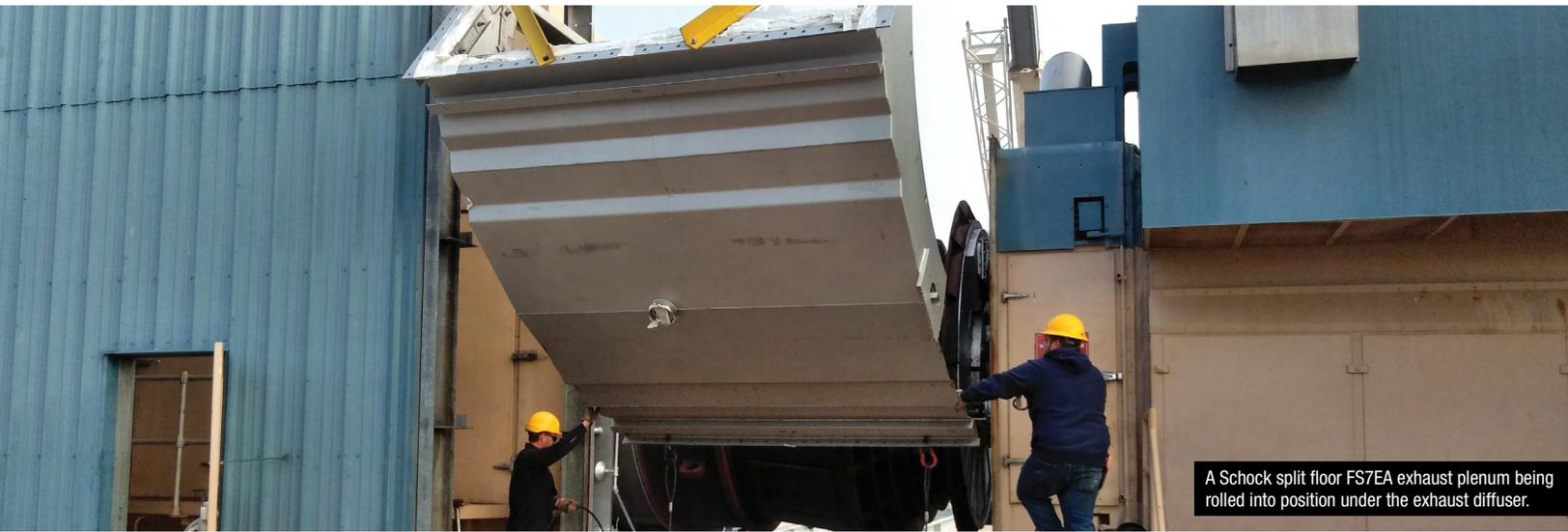
A Schock split floor FS7EA exhaust plenum being rolled into position under the exhaust diffuser.
