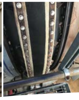
FS10D exhaust diffuser expansion assembly upgrade.
