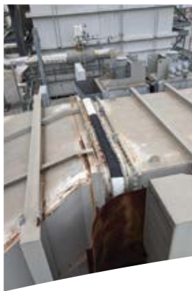
Exhaust expansion joint belt repair.
