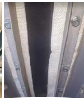
FS7F aft exhaust diffuser expansion assembly upgrade.
