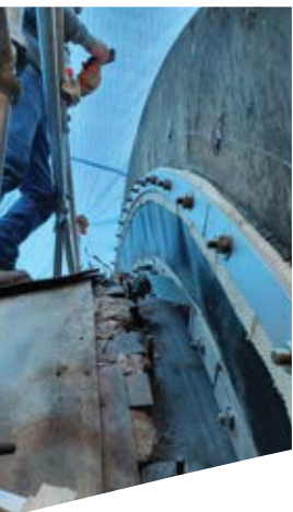
FS7F forward trough expansion joint.
