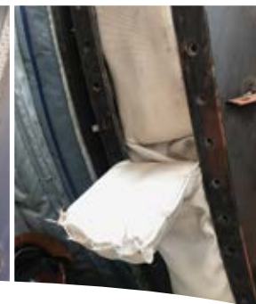
Installation of thermal protective pillows.
