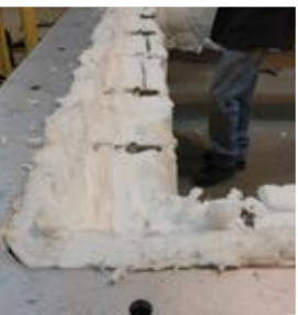
Expansion joint frame, ready for liner installation.
