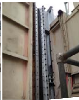
FS6 exhaust plenum expansion joint assembly.
