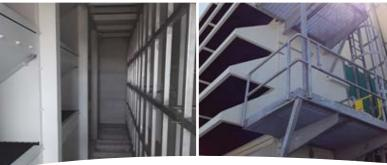
Rugged stainless steel filter grid construction to ensure positive filter element seal.
