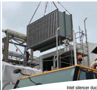
Inlet silencer duct installation (FS7EA)
