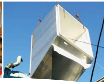
Externally lined inlet transition (FS7B)
