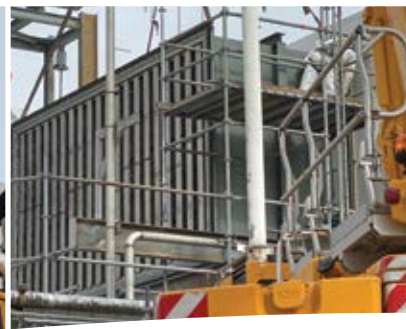
Inlet silencer duct installation (FS7EA)
