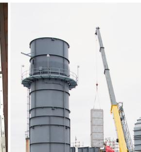
Installation of upgraded silencer panels for FS7F.
