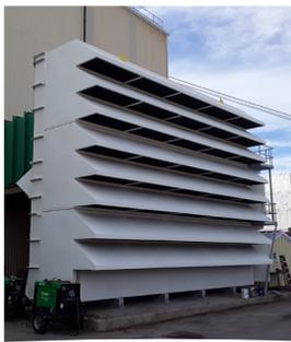
A Schock barrier filterhouse for a FS7E.
