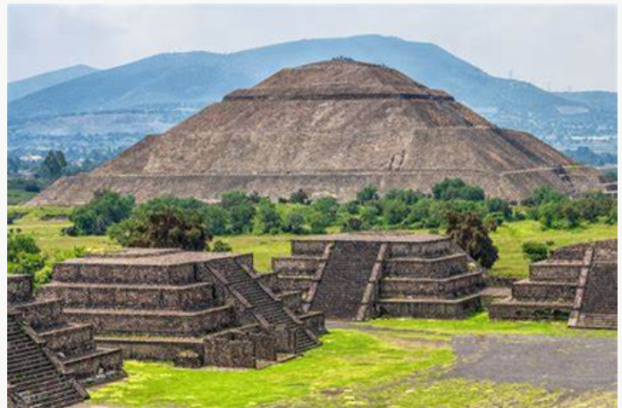
MicroPoz is used to repair the Meso-American pyramids and structures.
