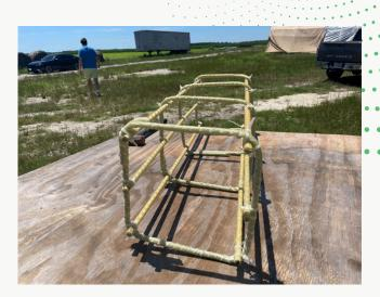
E3 was contacted by a builder looking to design and build TREBAR columns for a pool bar
