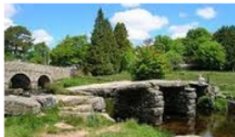
The Old Clapper Bridge, Postbridge
