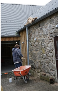
Harry pointing the walls of the shippen
