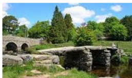
The Old Clapper Bridge, Postbridge
