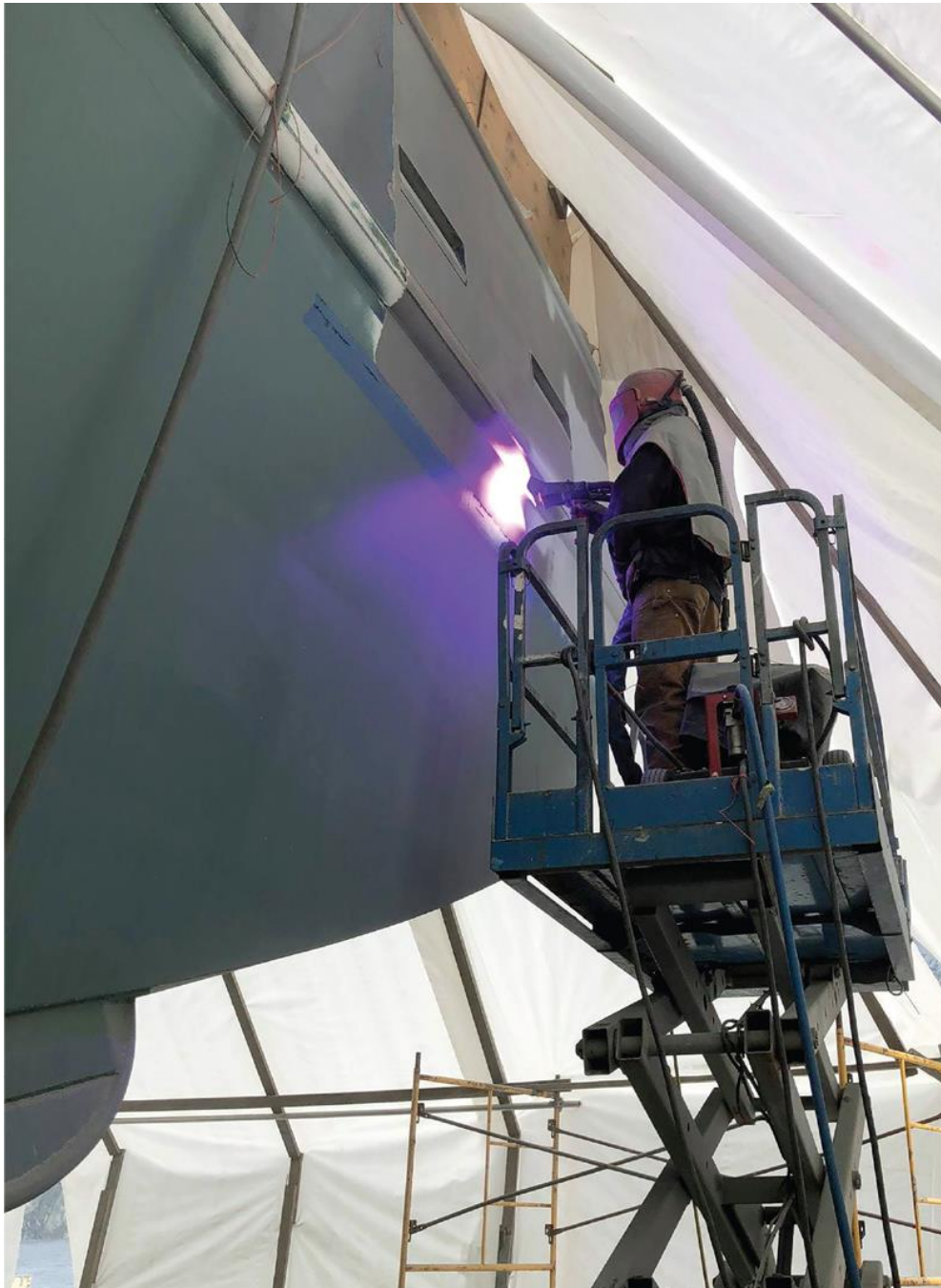
FIG. 1: Instead of shipping individual items off-site to be galvanized, the fabrication company was able to metalize structures in the field with in-house staff. Photos courtesy of the authors
