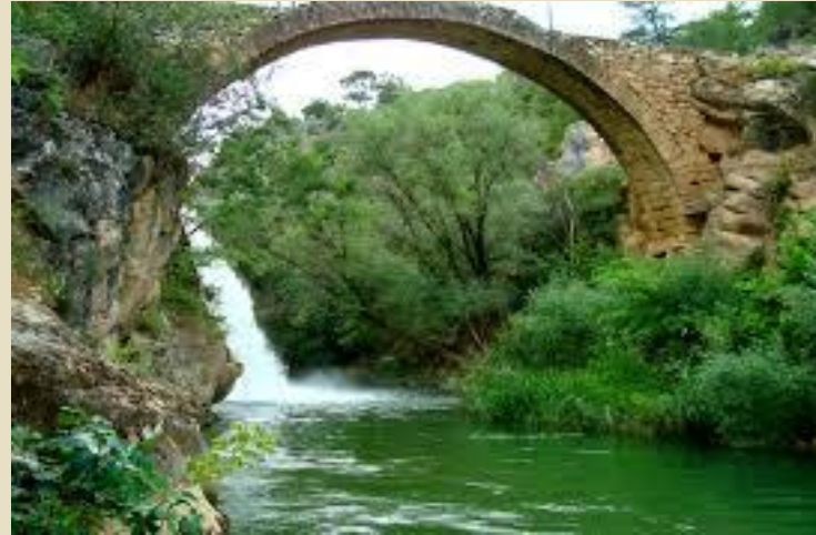
Karahallı Clandras Bridge
