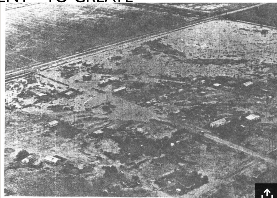
An aerial view of Allenville, a historic Black community south of Buckeye in Arizona's West Valley from 1944 to 1978.
