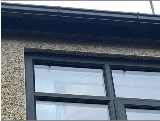
Photo - 9 UPVC roofline joinery
