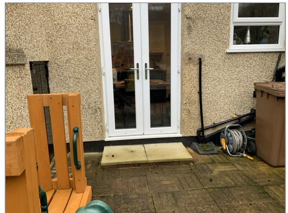
Photo - 8 Patio doors to rear
