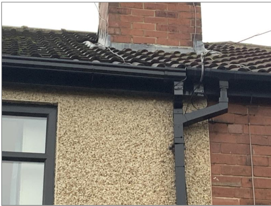
Photo - 4 Rainwater pipes and gutters
