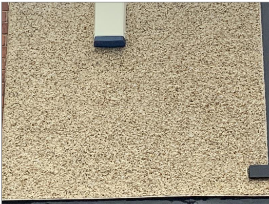
Photo - 5 Typical outside wall surfaces
