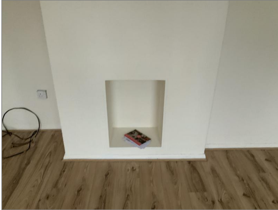
Photo - 15 Decommissioned fireplace
