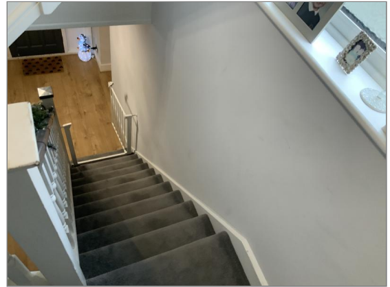
Photo - 18 Timber staircase
