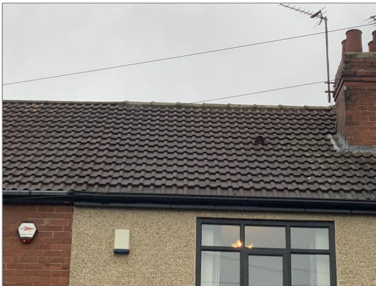
Photo - 3 Main roof coverings
