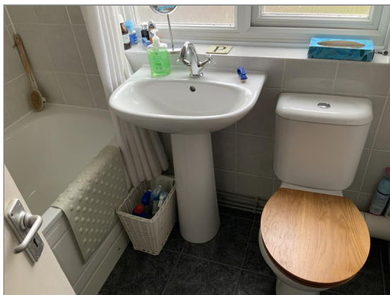
Photo - 19 Bathroom fittings
