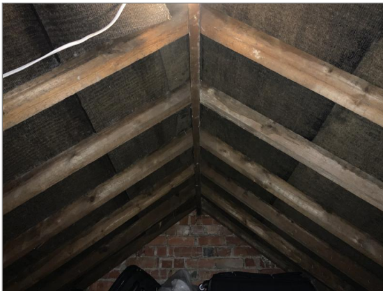
Photo - 10 Roof structure
