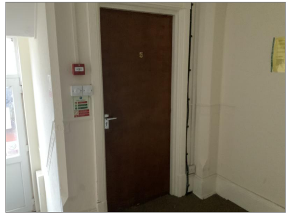
Photo - 31 Typical internal joinery
