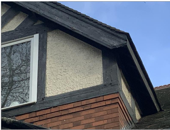
Photo - 15 Exterior joinery
