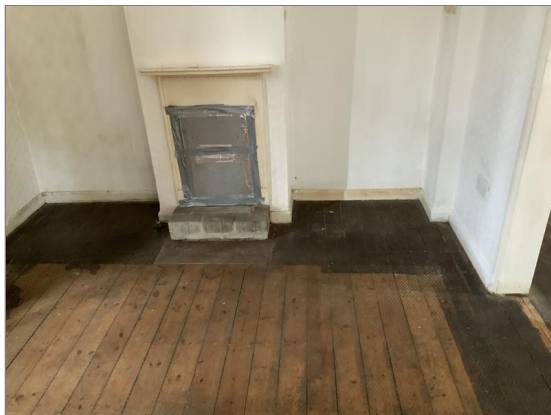
Photo - 26 Decommissioned fireplace
