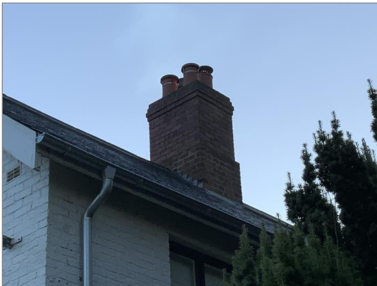
Photo - 2 Main chimney stack
