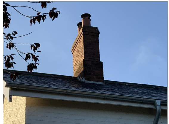
Photo - 3 Rear subsidiary chimney stack
