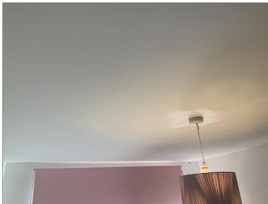
Photo - 19 Typical ceiling
