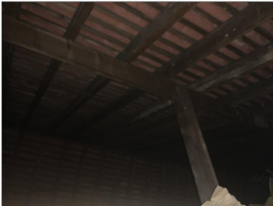
Photo - 18 Roof structure
