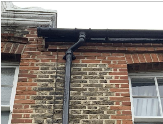
Photo - 7 Rainwater pipes and gutters
