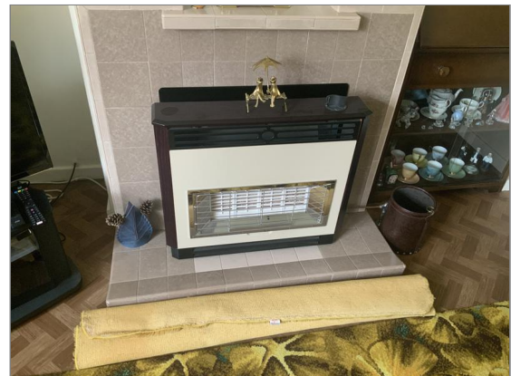
Photo - 27 Gas fireplace
