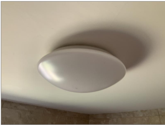
Photo - 32 None IP rated light fitting
