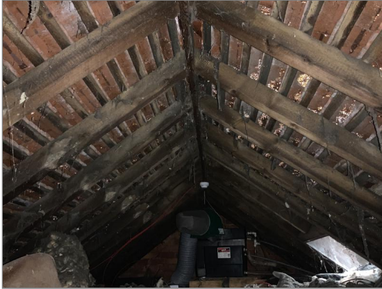
Photo - 16 Main roof structure
