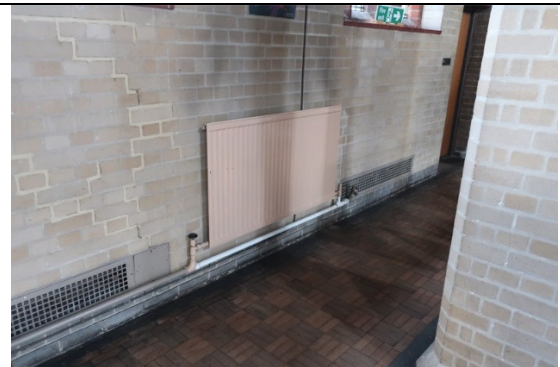
Radiator between two convactor grilles
