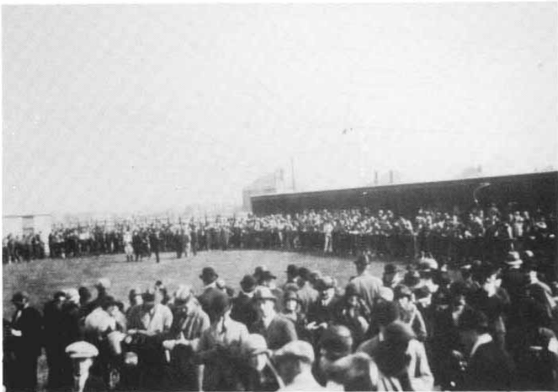
14. The Paddock (Western Avenue houses in the background).
