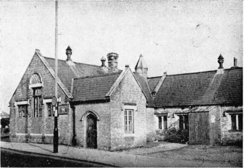
The original Kinson School before demolition
