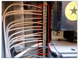
5.3 Item 1(Picture) Copper 15/20 amp branch circuits. 5.3 Item 2(Picture) Copper 15/20 amp branch circuits.
