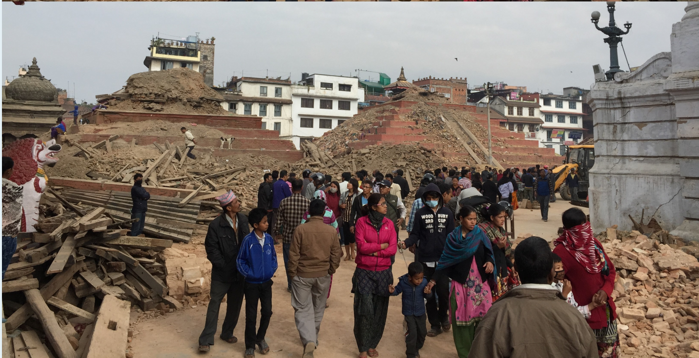
Collapse of National Monuments and houses in Kathmandu
