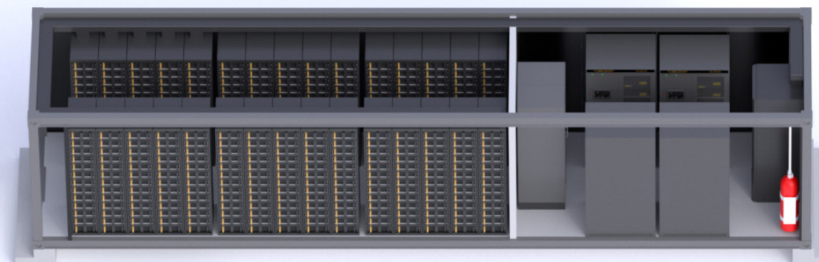
40ft ESS - CPT container
