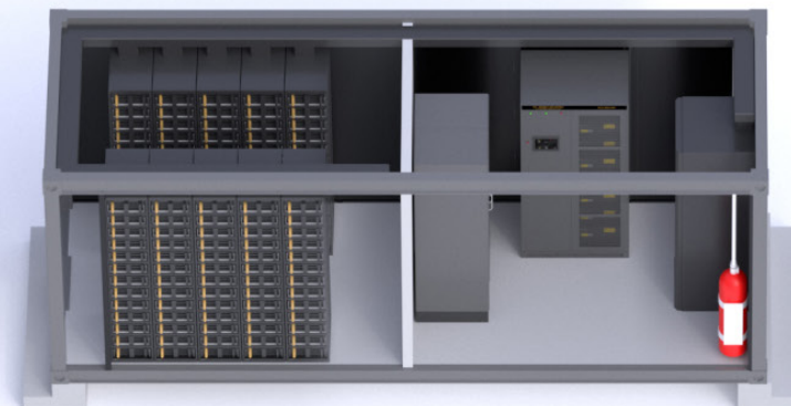
20ft ESS - CPT container
