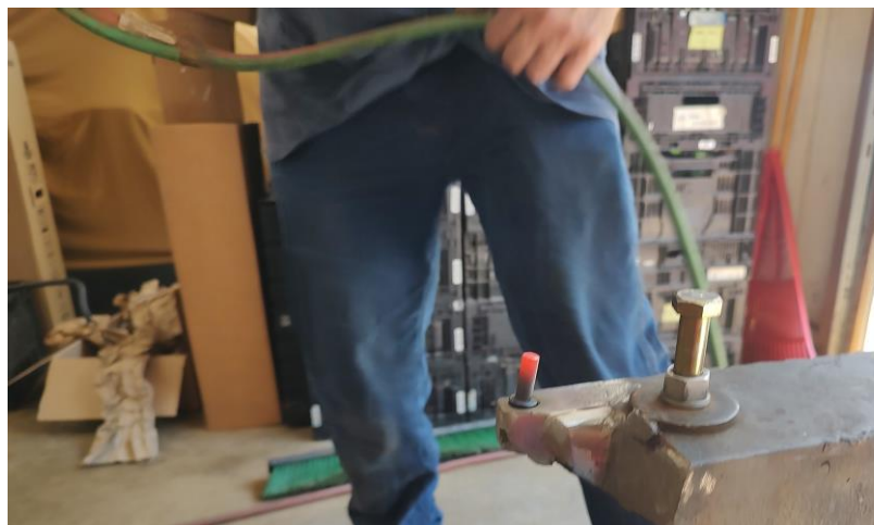
Figure 6 - Red hot rivet ready to be hammered in place
