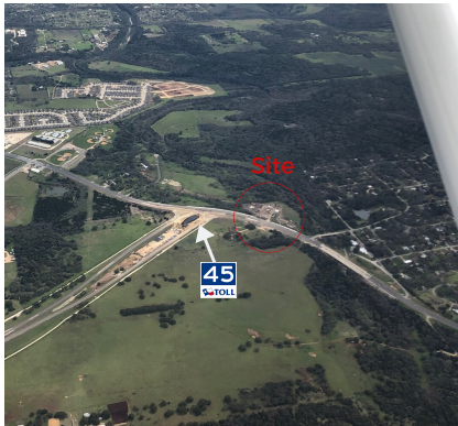
Aerial of SH 45 and Site
