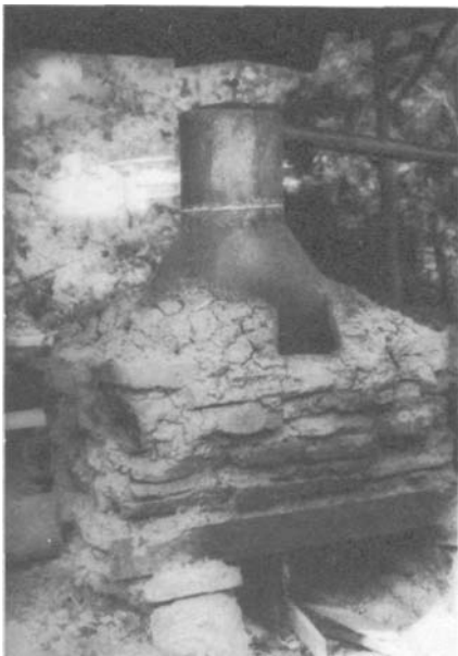
PLATE 263 A furnace made of rock and red clay. A fire has been started in the firebox, the cap has been sealed on with rye paste, and the operation is ready to go.
