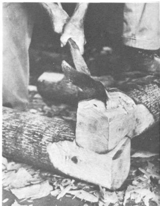
PLATE 73 Now slope the top log as before and raise a third log into place and duplicate the process just described.
