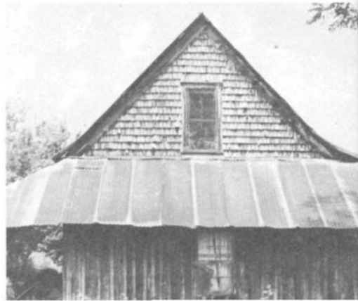
PLATE 117 A gable covered shingle fashion on a house near Franklin, North Carolina.
