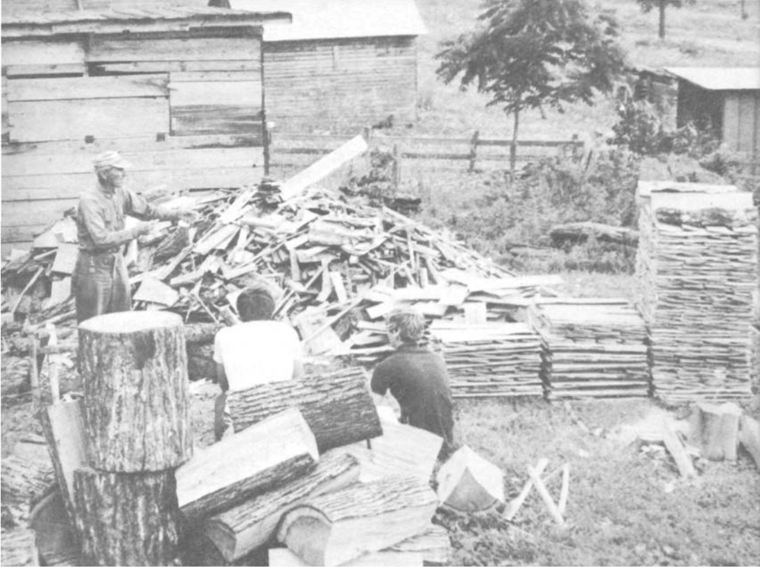
PLATE 33 The finished board is thrown aside to be stacked later. Often it took nearly five thousand of these boards to cover a large barn of about forty feet in length. A good board maker, however, could rive over a thousand boards a day if he kept at it steadily and didn't have to "bolt them up." If the boards have a slight twist, they can be "bumped," or the high places shaved off with an axe. Bill is making the boards in this photograph for Roy Thompson who is building a log cabin. (See next chapter.)
