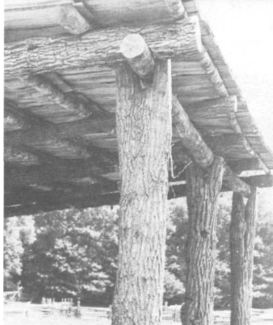
PLATE 103 A rough outdoor shed in the reconstructed pioneer settlement. The two plates are held by forked logs driven into the ground.
