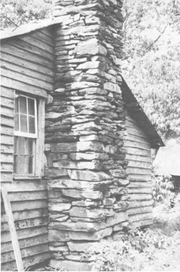
PLATE 143 A simple rock chimney chinked with red clay on a house near Toccoa, Georgia.
