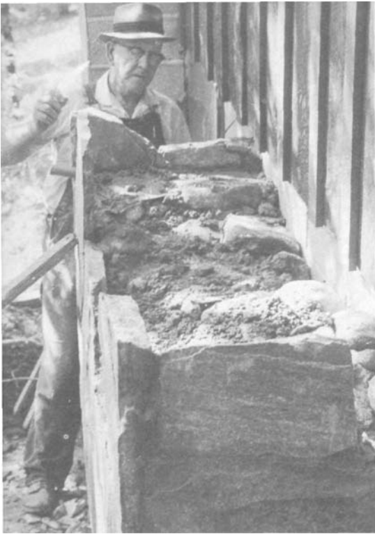
PLATE 148 Claude Darnell, a master chimney builder, often faces his chimneys with flagstone. The flagstone is cemented in place a round at a time, and the box thus created is filled with a "stuffing" of creek rocks and cement.
