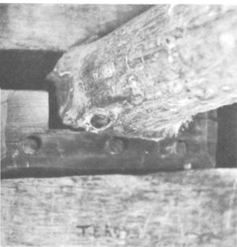
PLATE 102 The joists in this building rest in cradles pegged to the inside wall.
