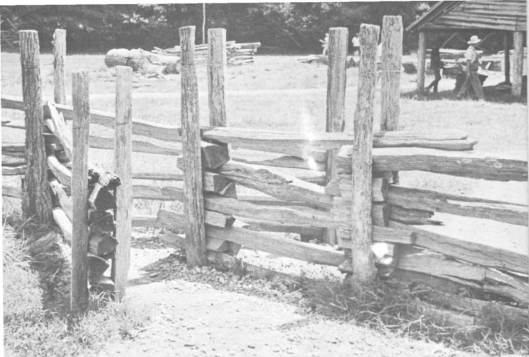
PLATE 6 A split rail fence in the reconstructed pioneer settlement at the Cherokee, North Carolina, entrance to the Smokies. The "V"-shaped opening eliminates the need for a gate that opens and shuts.
