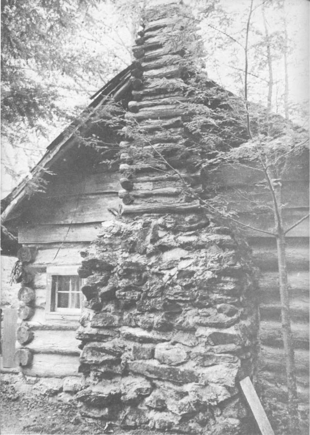
PLATE 145 A stick and mud chimney on a cabin near Highlands, North Carolina. Sticks were used only above the firebox which was of rock.
