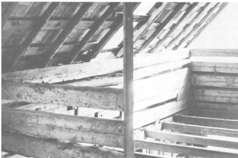
PLATE 94 The loft in this building rises five feet above the joists. Note the inside wall in the foreground.
