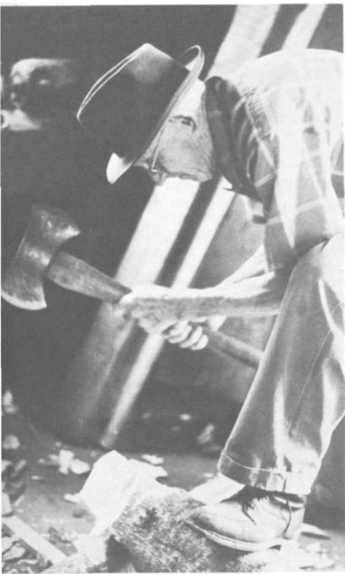
PLATE 81 Harley Thomas demonstrates another method for cutting the same notch. Hew a peak as above.
