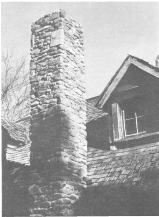
PLATE 150 Another example of Claude Darnell's work. This masterpiece, a flue for a furnace, is on the weaving shed at the Jay Hambidge Art Foundation in Rabun Gap, Georgia.
