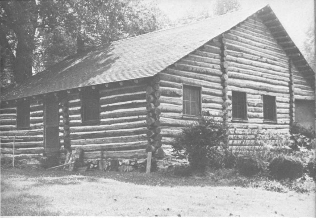
PLATE 126 The Happ'n'so house has pole laths that are really only two feet long and serve only to help support the gable logs and the overhang. The house has a full set of pole rafters.
