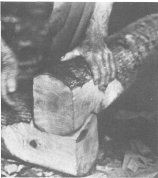
PLATE 72 Place the two together and check the fit. If not perfectly snug, shave off the high places using the axe as a chisel . To make the top log fit farther down on the bottom one, cut the notch deeper while maintaining the same slope.
