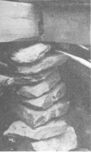
PLATE 44 A foundation pillar made of rocks placed atop each other.
