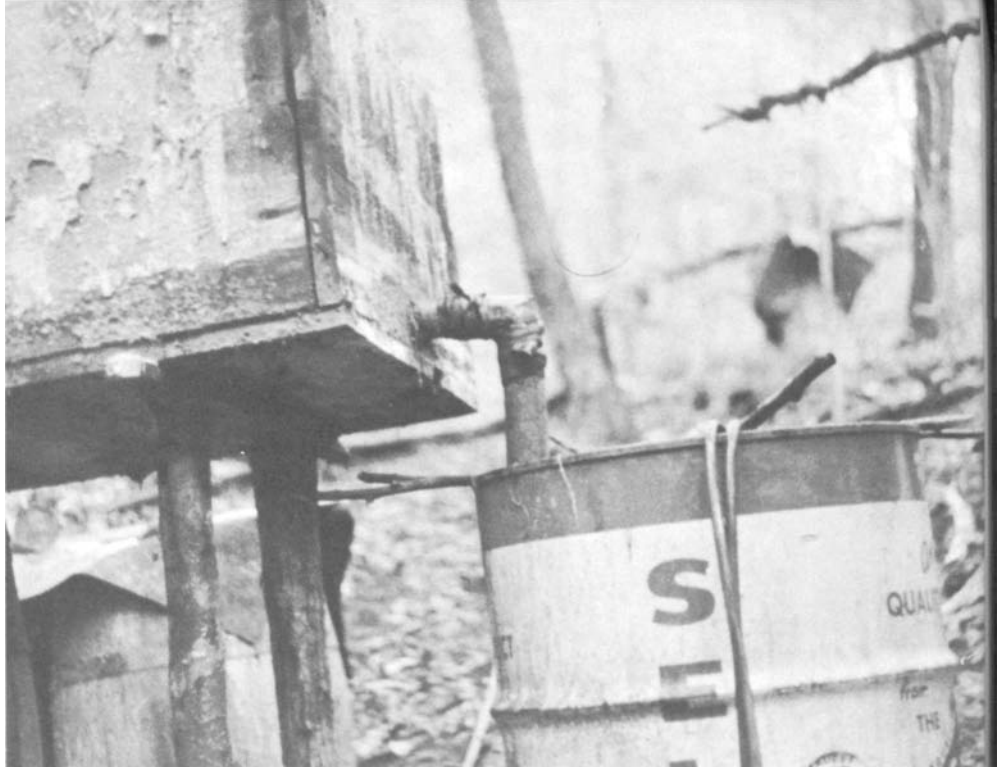
PLATE 275 The heater box from the other side, showing the connection between the heater box and the condenser which is mounted in the metal drum.
