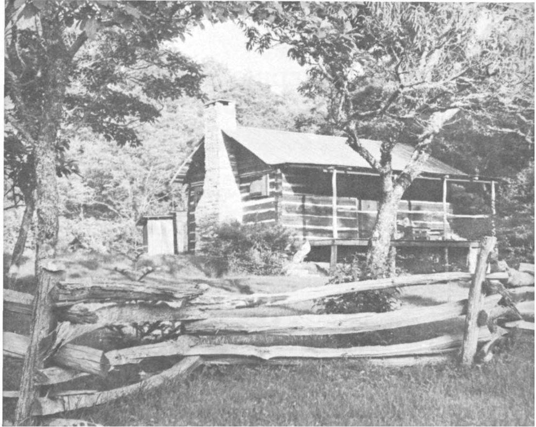
PLATE 39 This building near Highlands, North Carolina, shows why one might still take the time to build a log cabin.
