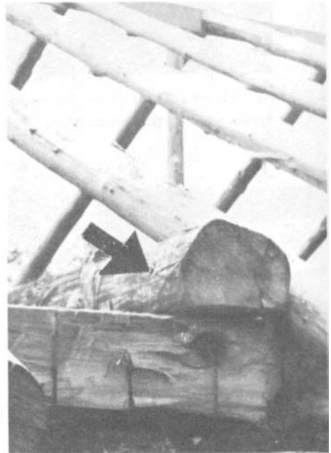
PLATE 98 Note how the joist (arrow) is left round except for the lap joint cut to fit the plate.
