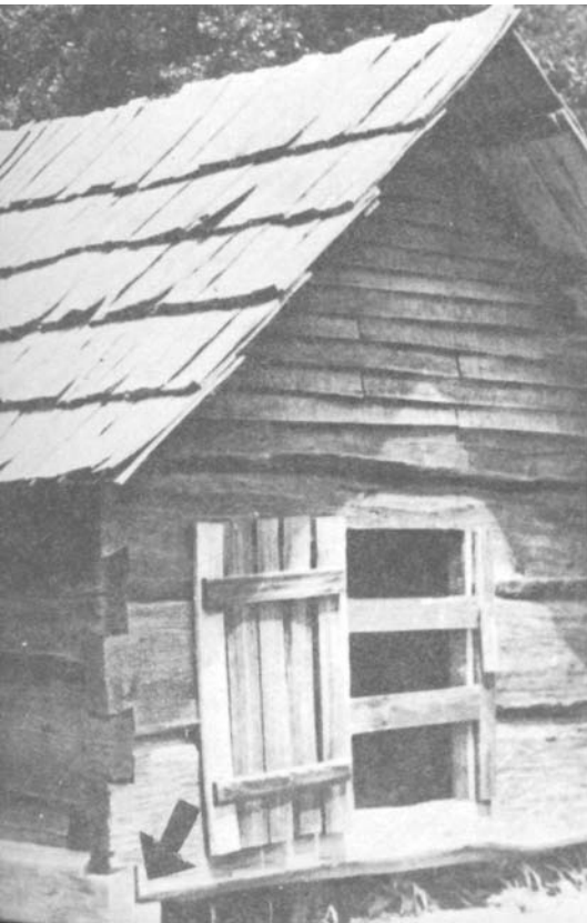
PLATE 48 In this building, part of the pioneer settlement, the sill is quarter-notched (arrow and Plate 49).
