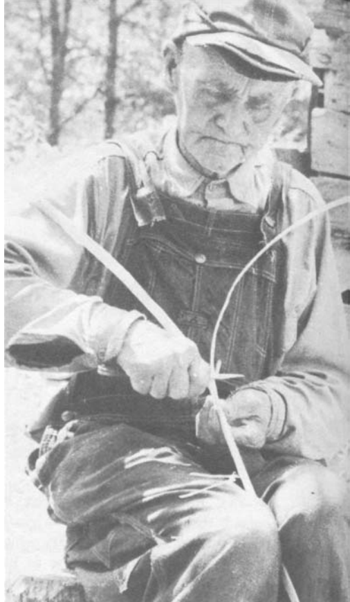
PLATE 157 If one edge binds or catches while the splits are being pulled apart, it can be freed using the knife.
