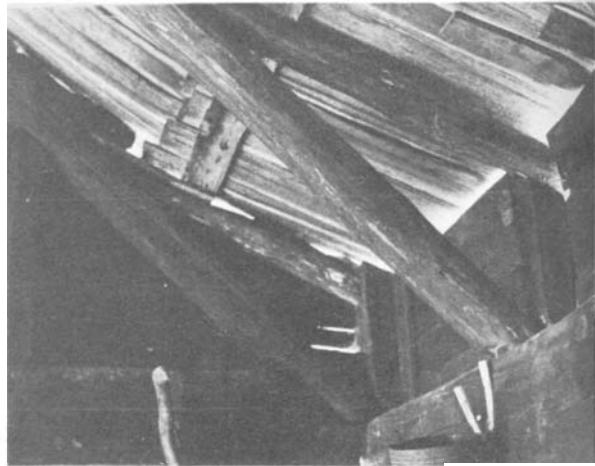
PLATE 114 Both house and porch rafters are visible here. The same scheme is diagrammed in Plate 115.
