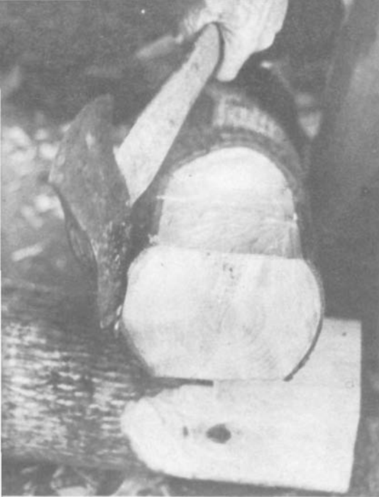
PLATE 70 Now hew out the outlined area of the top log. Hew to the line.
