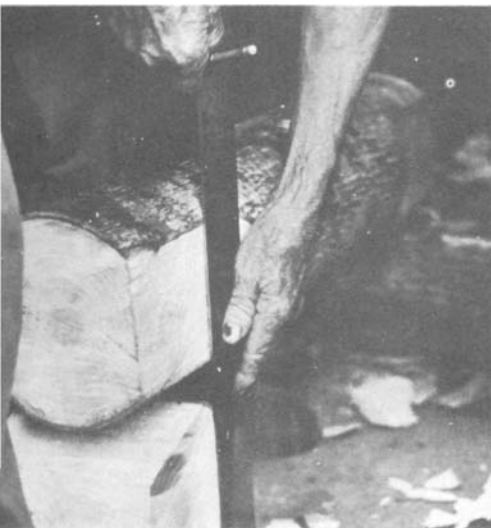
PLATE 68 Now, placing the ruler as shown, draw a vertical line on the top log which intersects with the sloping line.
