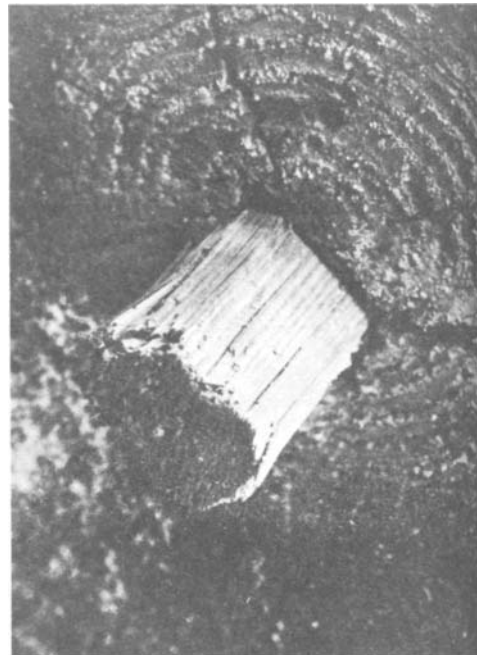
PLATE 134 A locust peg over two hundred years old in the hole it was cut to fit.
