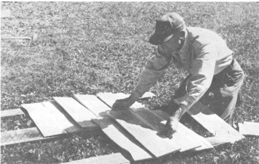
PLATE 34 Bill shows how the boards can be mounted on a roof.
