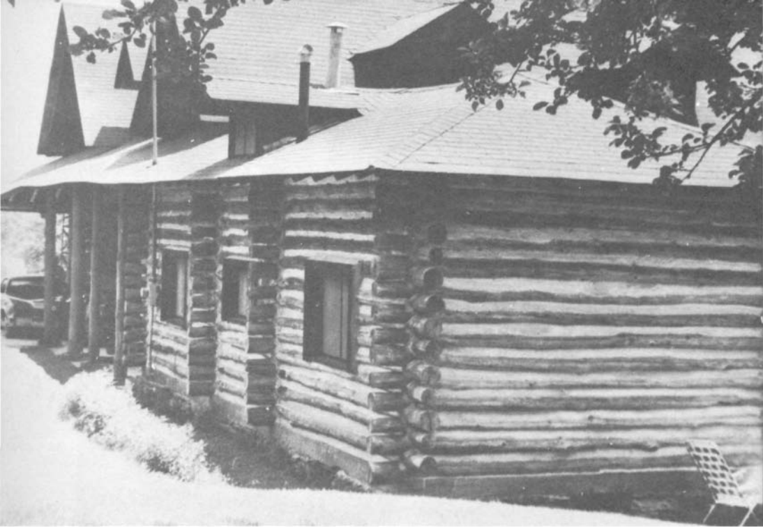
PLATE 91 The ends of the inside partitioning walls are clearly visible in this house, located on Dog Mountain near Highlands, North Carolina. Harley Thomas helped "notch up" this house in 1926 for Colonel Sewell who died not long after the house was finished.
