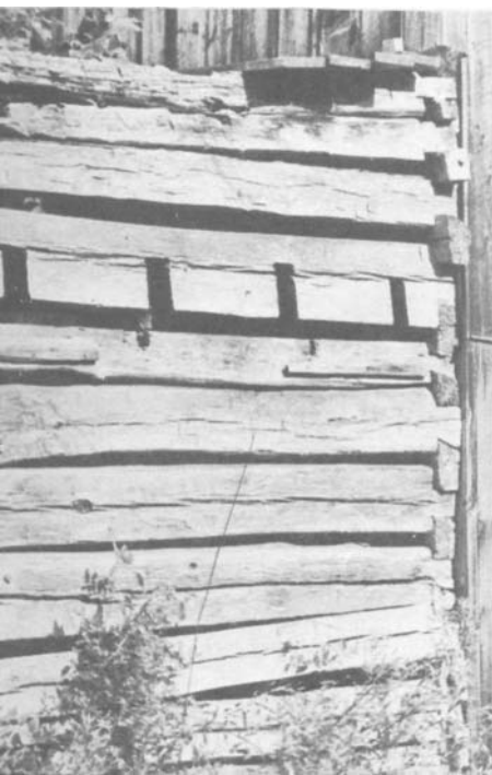
PLATE 95 In this building south of Franklin, North Carolina, the underside of the plate has been notched to accommodate each joist. Note the logs added above the plate to form a loft.
