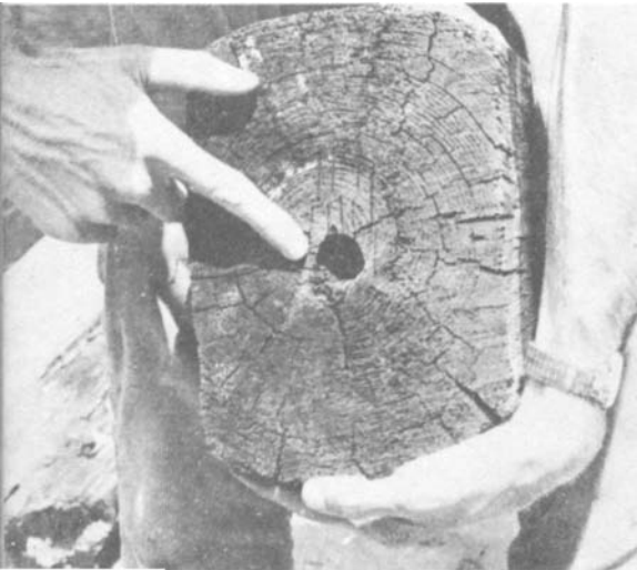
PLATE 133 A hole, drilled with an auger, into which the peg through the doorframe will fit.
