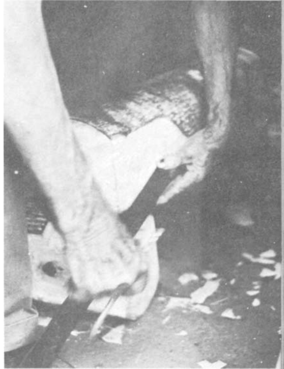
PLATE 67 Rest a steel ruler on the slope of the bottom log, and draw a line along the top edge of the ruler onto the side of the top log.
