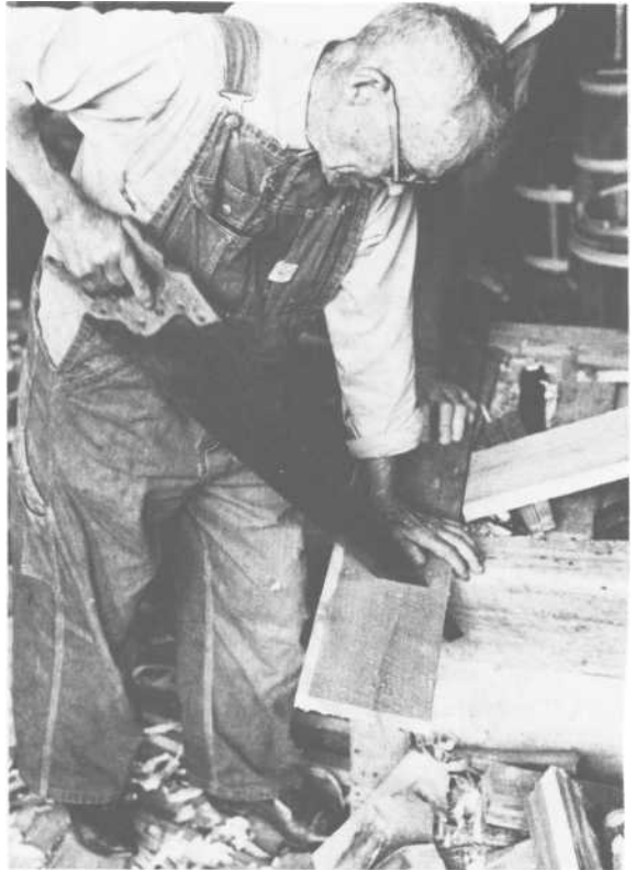
PLATE 357 Cut off the board piece with a handsaw.
