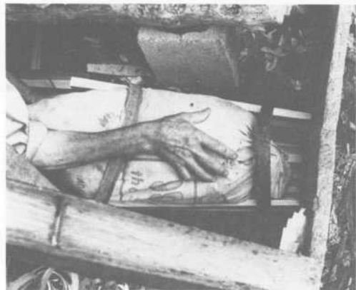
PLATE 345 Alex pushes a straw-filled bag between the hoops to hold the shape as the staves are added.
