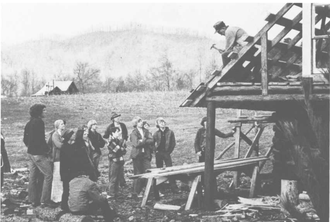
PLATE 312 A group of Foxfire editors watch as Woodrow nails on row after row of 24" long hand-split white oak boards. He is placing them on board fashion (see Plate 315 ).
