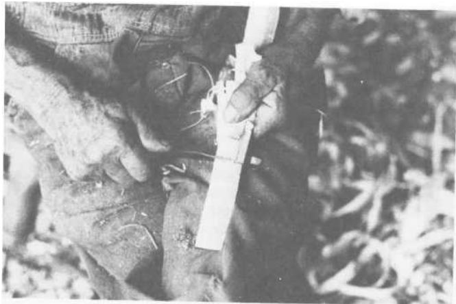
PLATE 375 Step 18: Begin to shape one hoop end with a pocketknife; the hoop end is shaved as it is shaped. Each hoop will eventually fit around the churn and the ends will fasten together.
