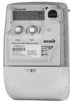
Figure 6.1: A smart meter
