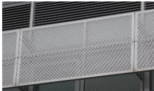
Figure 7-2 Fine metal mesh on building surface
