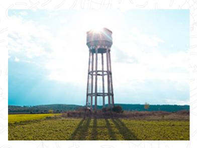
and those pumps don't need to run all the time. They can run only when needed. Which means that this can work in an intermittent power grid failure situation. In other words, if your power grid is only working one hour a day, you can use that hour to pump water uphill into the tank, and then for the next 23 hours, let's say, you have water pressure. You don't need a pump that has on demand pressure constantly every time somebody is using water.
