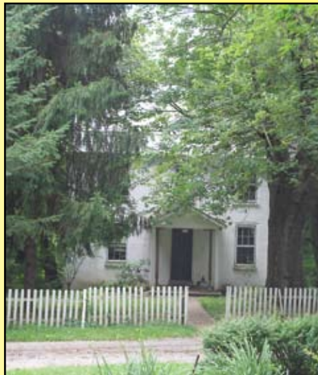
The tenant house on the McKean property.
