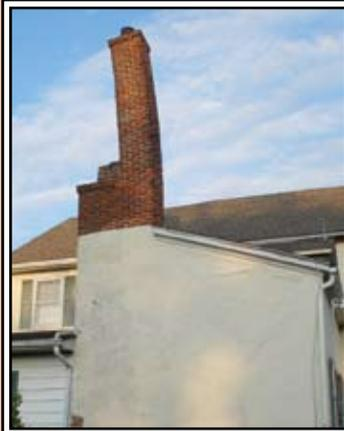
Side view of the original log dwelling shows the crooked chimney. It is thought an extension of the original chimney was needed after the additions.
