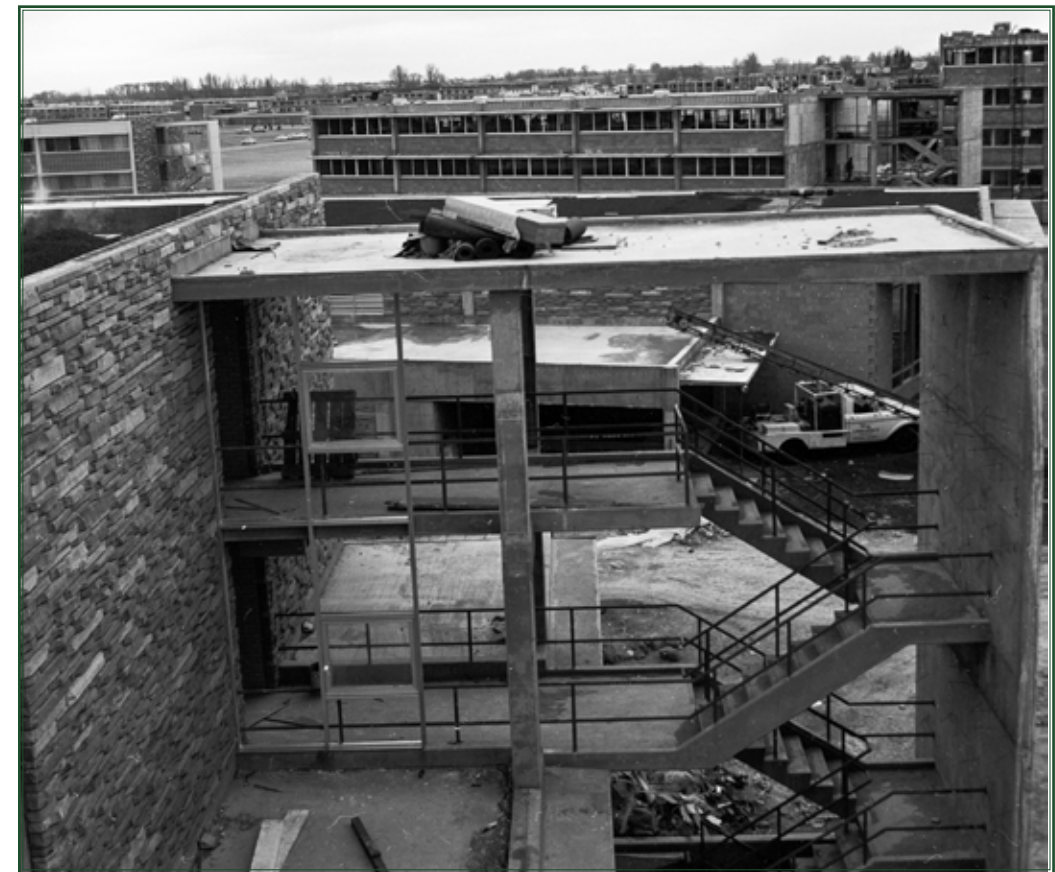
A stairwell between wings under construction. Circa 1964
