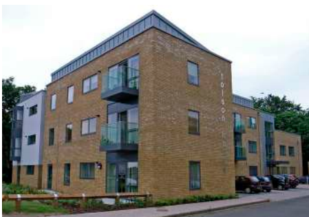
Residential, North Street.
