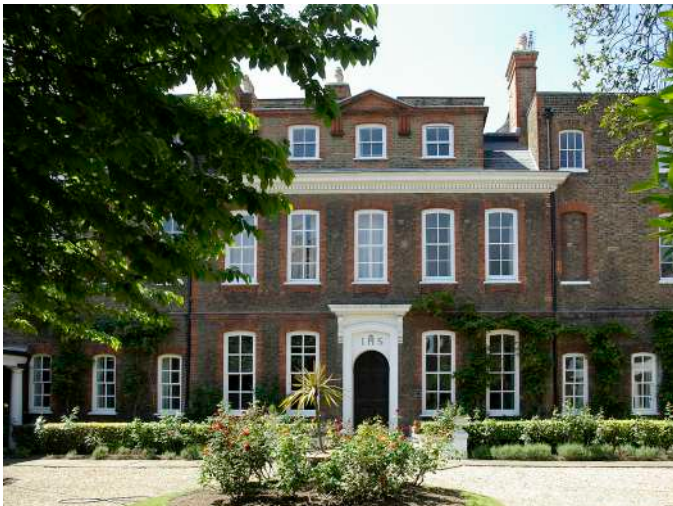
Gumley House, Twickenham Road
