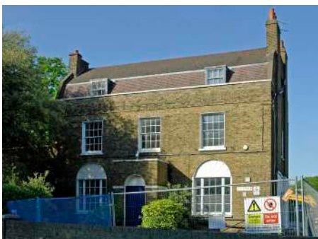
Busch House, Twickenham Road
