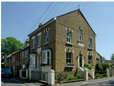
Locally listed May's Villas, Byfield Road
