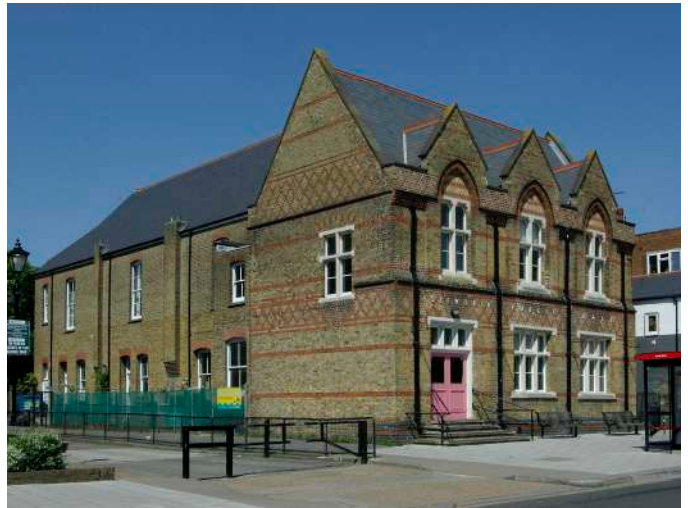
Isleworth Public Hall, South Street
