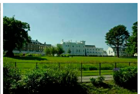
The Grounds of Isleworth House.
