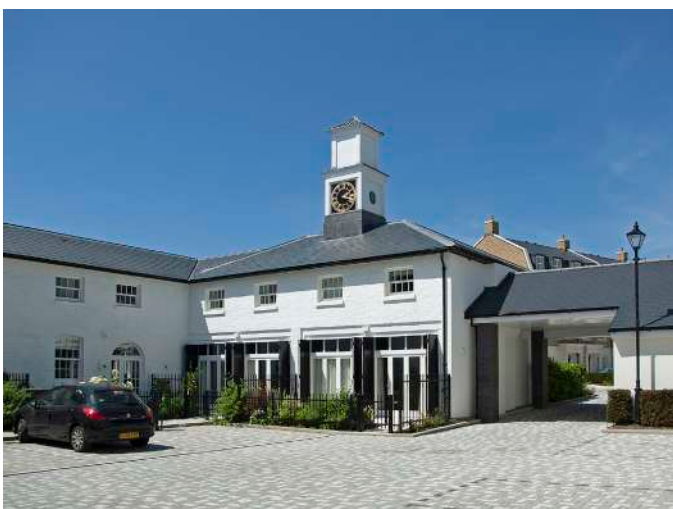
Redeveloped stables courtyard with clock turret.
