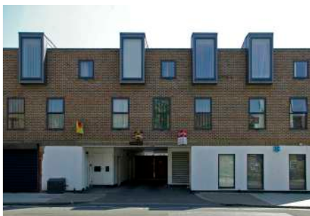
Residential, South Street.
