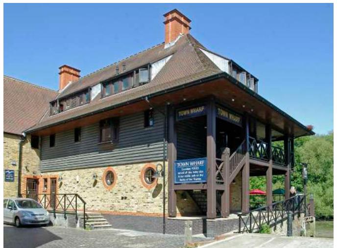
The Town Wharf public house, Swan Street
