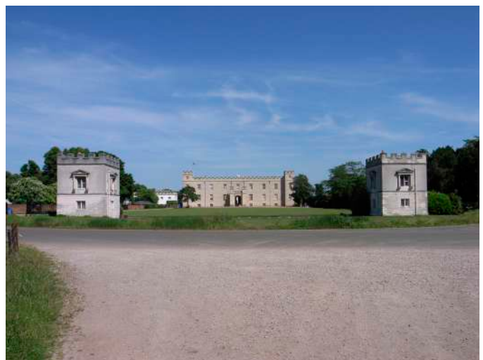
Formal view of Syon House and the two lodges.
