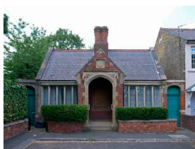
Grade II Listed Butler's Almshouses, Byfield Road
