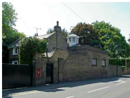
Rear of Redlees cottage, Worton Road
