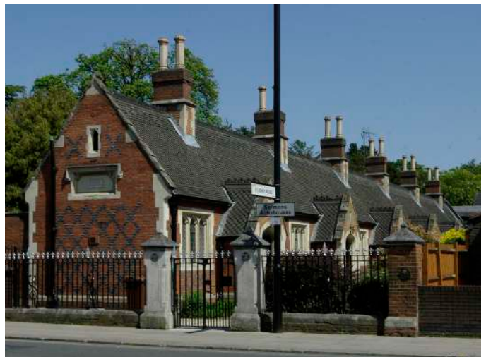
Sarah Sermon's Almshouses, corner of North Street and Twickenham Road
