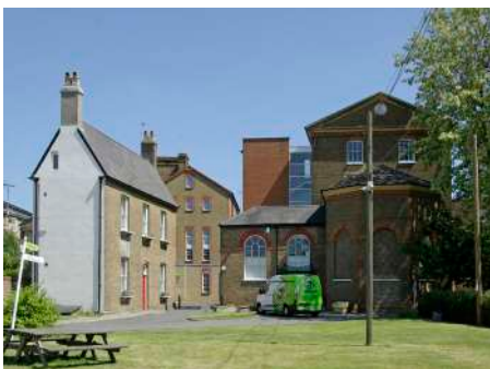
Rear of Gumley House, Twickenham Road
