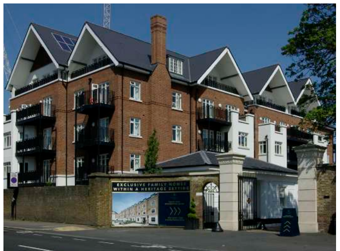
The wall, gate and lodge with new housing behind.
