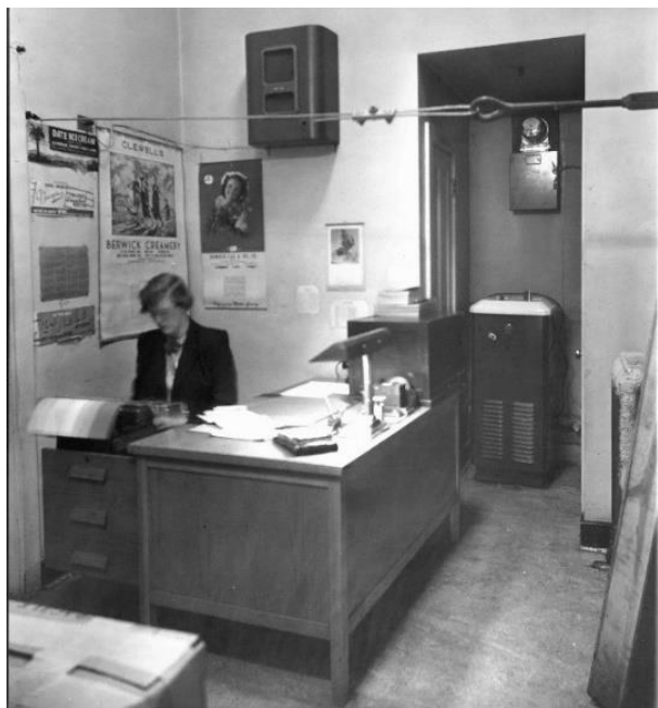
PRIOR TO RENOVATION OF THE WOOLWORTH BUILDING TENSION WIRES KEPT WALLS FROM SEPARATING
