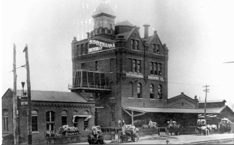
Susquehanna Brewing Company Plant pre-1920 producer of the Stegmaier brand at Alden and Main Streets
