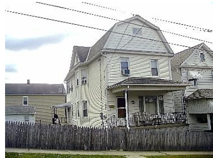
115 West Field Street
