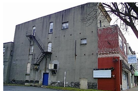
One can see the building's original version behind the added façade.
