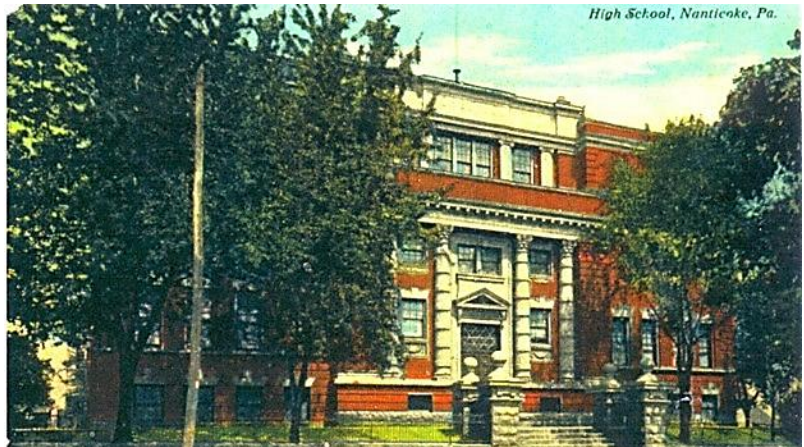
Pulaski High School Completed in 1906
