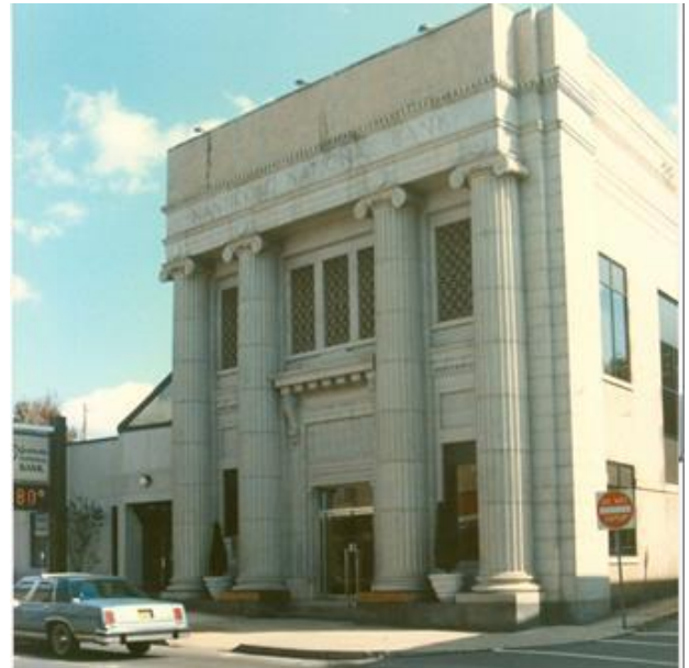
The Nanticoke National Bank added an addition in 2008 after the demolition of the Leader Store on Main Street.
