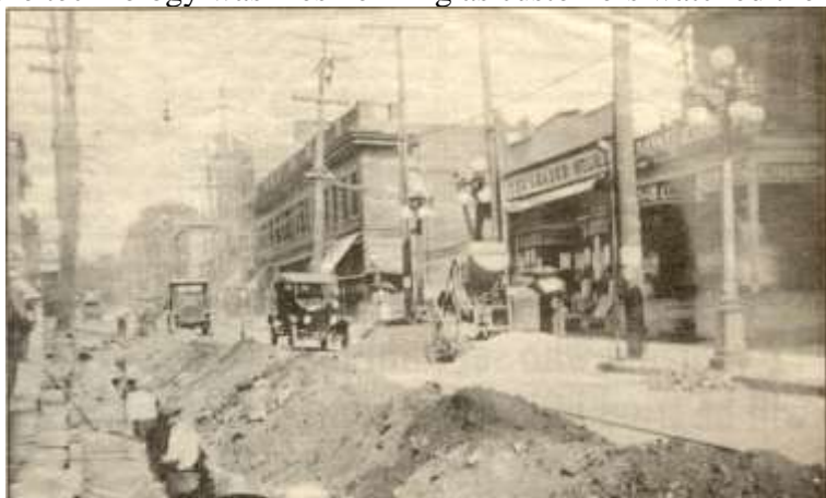
Work on Main Street is underway in front of the Leader Store in this undated photo
