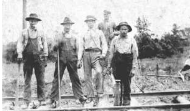
Peoples Street Railway Maintenance crew in 1912
