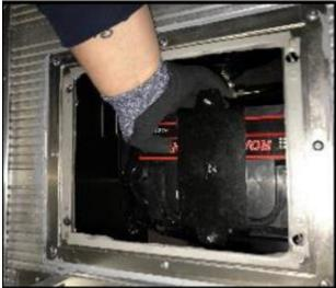
Use 7/16<sup>th</sup> wrench to loosen both nuts on tie down bracket
