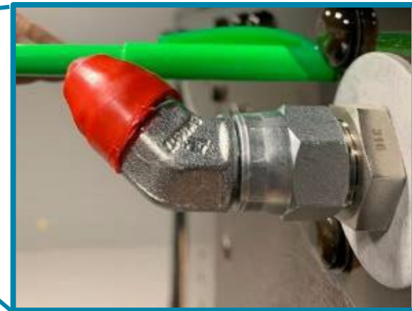
PRD vent outlet with PRD cap
