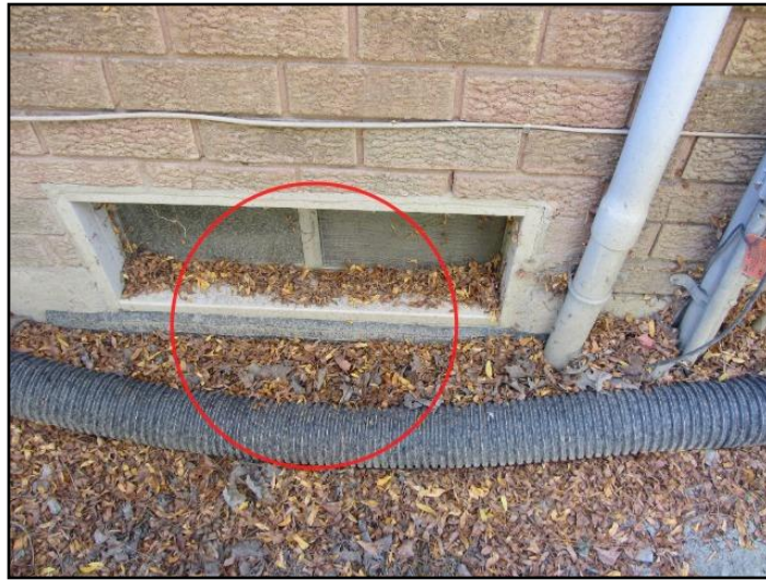
8. Less than 6 inches below window
