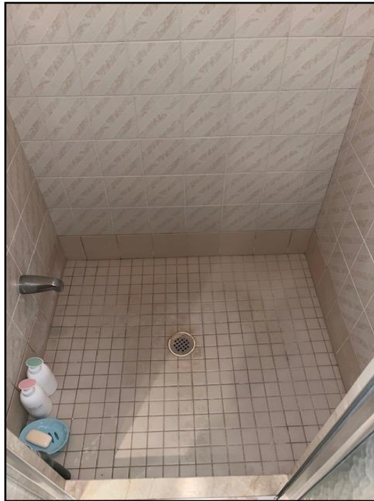
28. Caulking loose, missing or deteriorated
