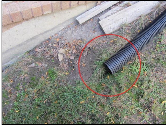
7. Discharge to close to the building.
