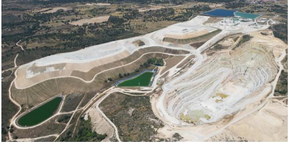
Barruecopardo Open Pit end of June 2024
