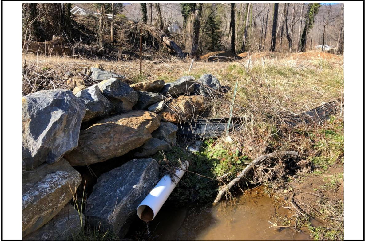
**PHOTOGRAPH 17:** A view of the unidentified pipe draining onto the subject property. The pipes source could not be verified as it originates on private property that is not associated with the subject property.
